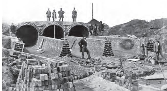
Joseph Bazalgette (top right) at the northern outfall sewer being built below London’s Abbey Mills pumping station. Photo Otto Herschan
